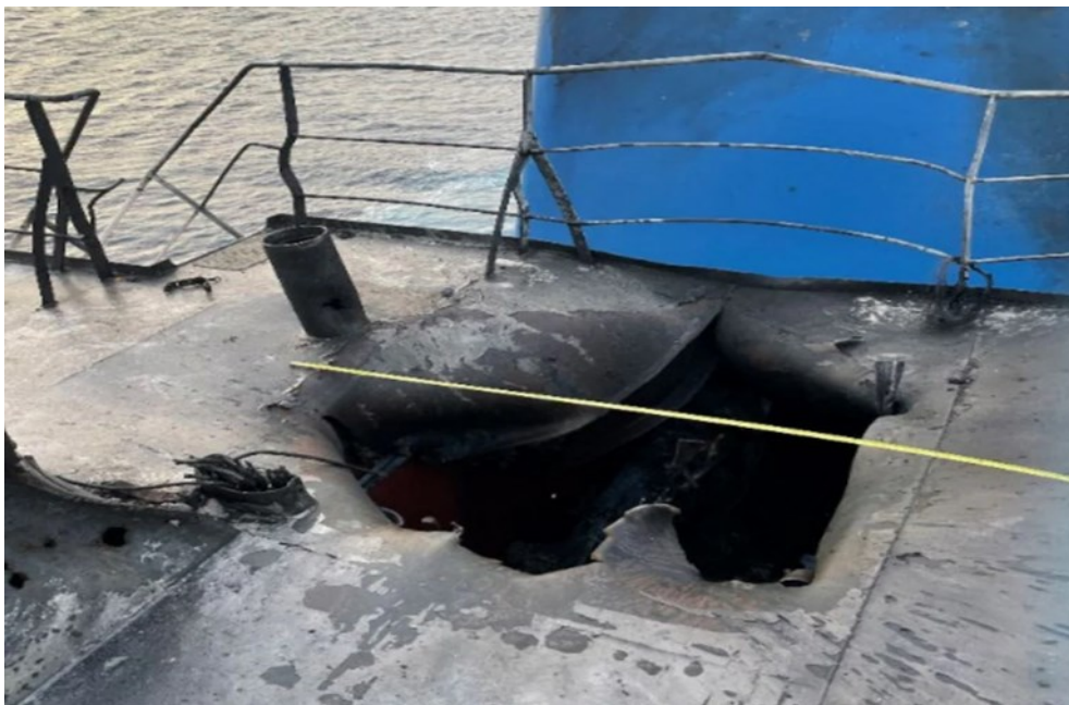
Figure 10. Damage Caused by a Drone Attack on the Oil Tanker (Mercer Street)
