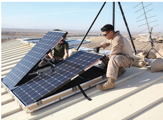
Figure 15: US Marine Corps troops installing solar panels on a combat outpost in Afghanistan (November 2012) to provide power to radios, laptops and computers. 72
