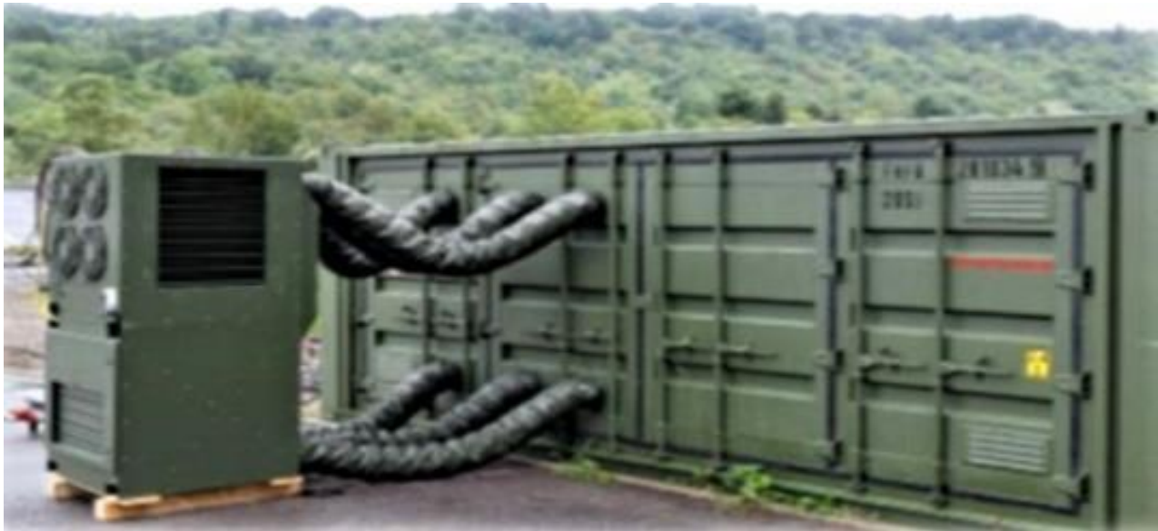
Figure 3. Transportable external HVAC module regulating temperature of battery container 20
