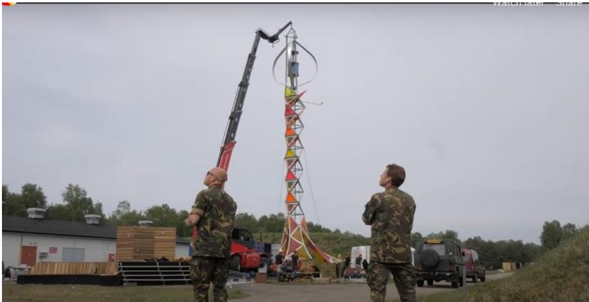
Figure 11. Netherlands military setting up GEM wind tower at Smart BaseLab 75
