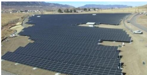
Figure 6. Existing base 2 MW solar array (1 MW connected to the test microgrid) that participated in the SPIDER tests 46 . This massive arrangement however is not an optimal size for a mobile camp where there is limited time and resources for extensive transportation/installation and dismantling..
