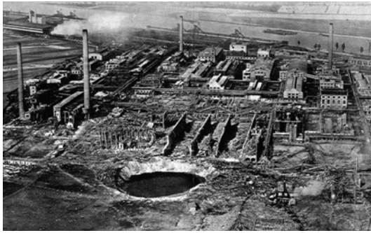
Figure 3: Aerial photo of the BASF Oppenau/Ludwigshafen (Germany) production plant after the devastating explosion of 400 tonnes of ammonium sulphate nitrate in 1921 causing 559 fatalities (Abelshausen 2003). The crater in the foreground indicates the location of the storage area where the explosion happened.
