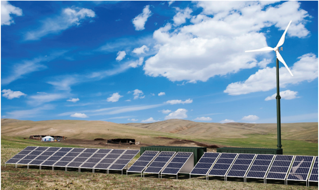
Figure 10: Deployable Modular Hybrid Power Generation and Management System designed within the NATO ENSEC COE's project
