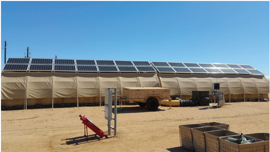
Figure 16: Fixed military installation equipped with solar panels. Basic expeditionary airmen skills training at Lackland Air Force Base in San Antonio
