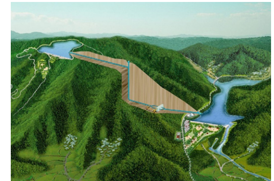
Figure 25. Bear Swamp Pumped Storage in South Korea
