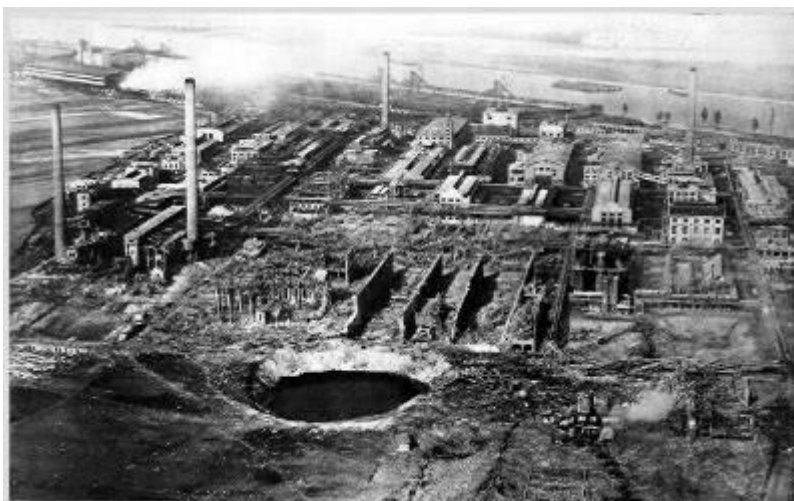
Figure 3: Aerial photo of the BASF Oppenau/Ludwigshafen (Germany) production plant after the devastating explosion of 400 tonnes of ammonium sulphate nitrate in 1921 causing 559 fatalities (Abelshauer 2003). The crater in the foreground indicates the location of the storage area where the explosion happened.
