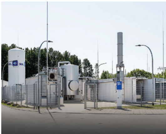
Figure 10: The Power-to-Gas Plant Falkenhagen in Brandenburg, Germany is operated by Uniper SE since 2012. Uniper was outsourced in 2015/2016 from the e.on AG, one of the former regional monopolists for electric power generation in Germany. The two containers on the right hand side of the picture hold the electrolysers. The left hand side shows the methanation unit for conversion of carbon dioxide into methane (uniper 2017a).
