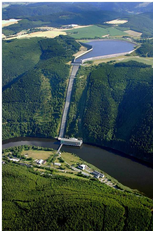
Figure 6: Pumped storage hydropower station Hohenwarte II in Thuringia, Germany which is owned by the Swedish company Vattenfall GmbH. The upper reservoir is filled with pumped water from the lower reservoir/river power plant in times of surplus electricity production. The water from the upper reservoir powers on demand the eight turbines in the machine hall, the height of drop is 304 m. 4,5
