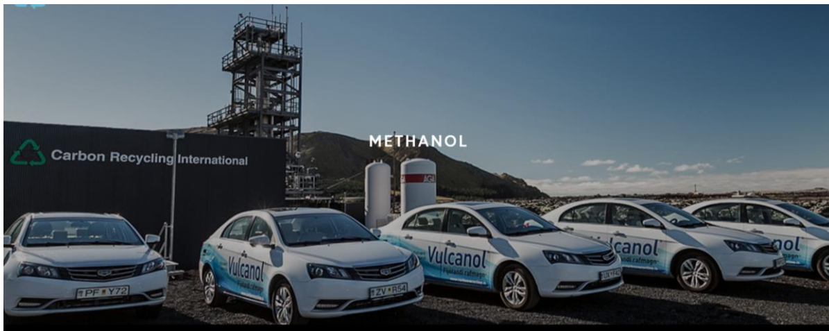
Figure 5: View of the Carbon Recycling International (CRI) plant in Iceland. The electricity is generated from geothermal sources. The carbon dioxide is captured from geothermal sources as well. Both raw materials are synthesised into methanol, which can be used as fuels in internal combustion engines (here as brand name “Vulcanol”), fuel cells and as chemical base material 19 .
