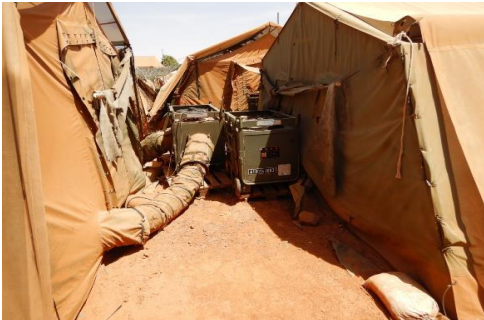
Figure 2: Inaccessible AC units
