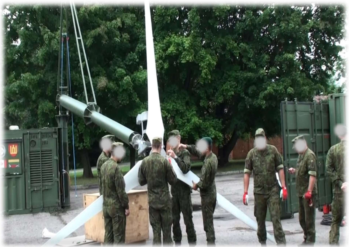
Figure 20. Wind turbine and its installation, Marijampolė, Lithuania (2018)
