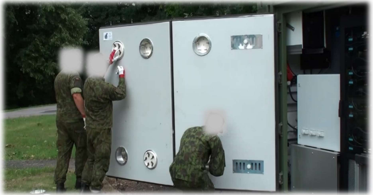
Figure 10. Training in Marijampolė (Lithuania): preparing HPGS cooling/heating module
