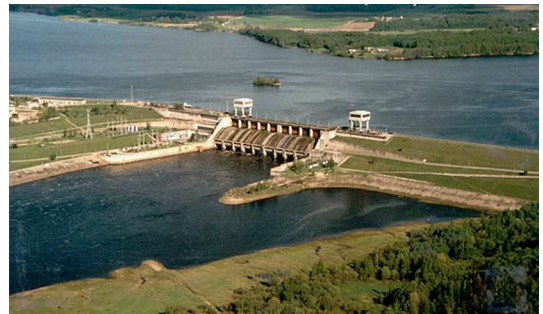
Aerial View of Plavinas HPP on the Daugava River
